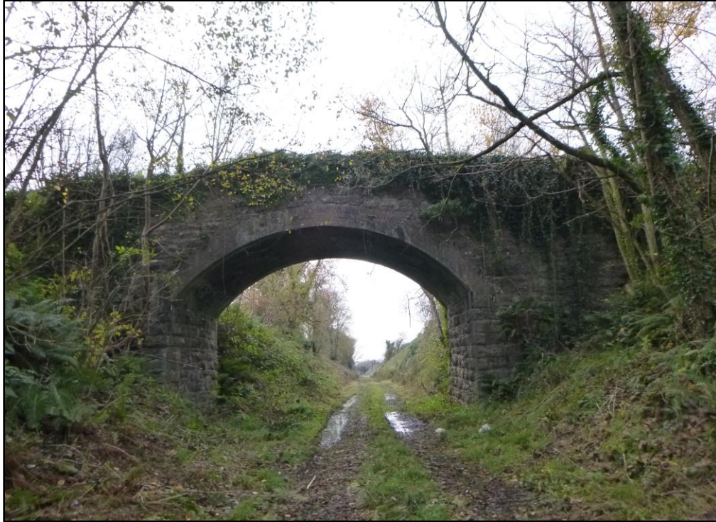
Plate 13 View WSW along railway cutting toward crossing point of The South – North Access Road; arched bridge carrying 18th century roadway that accessed the Newpark House area from the north (Shanarc Archaeology Ltd. 29.11.2023).
